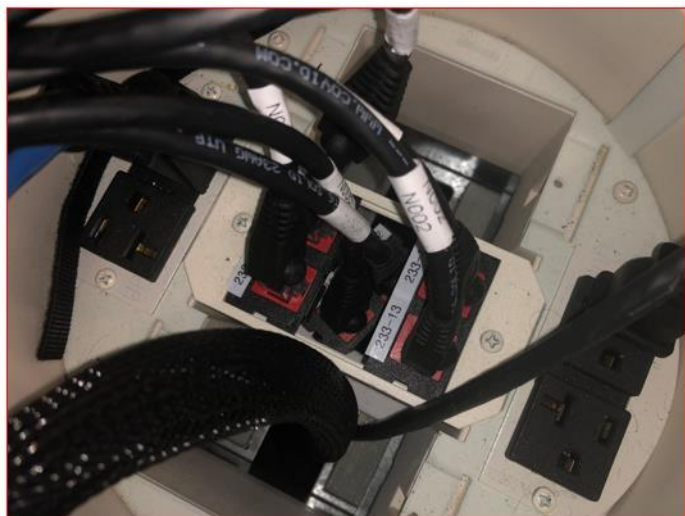
Not Acceptable: Floor box with unterminated cables passing through floor box.
