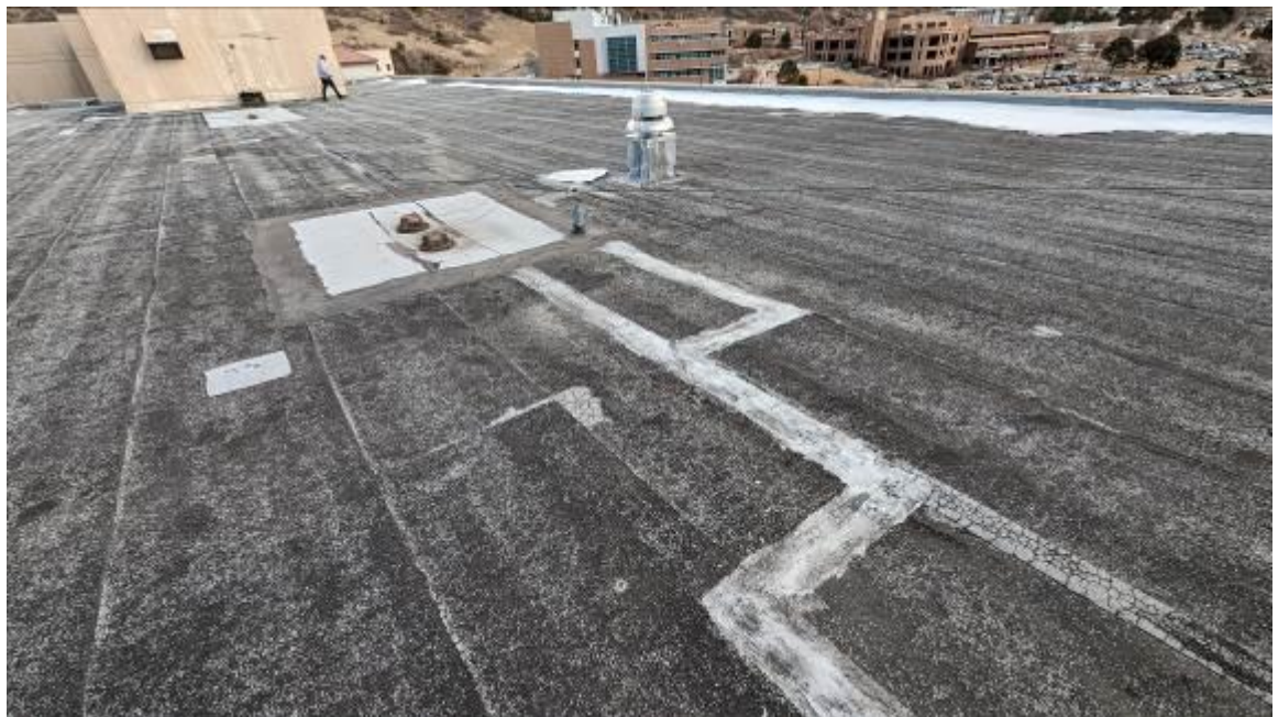
Silver coat on seam patches that came back with a Trace that was successfully point counted below 1%
