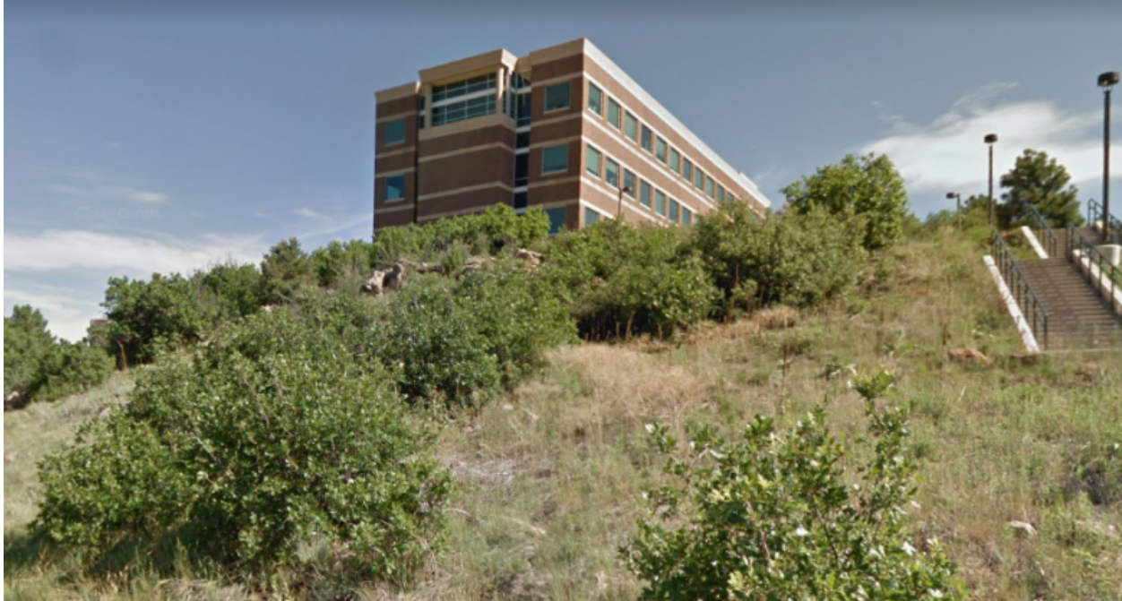
The slope of the land is everywhere at UCCS (picture is SE corner of Columbine Hall)
