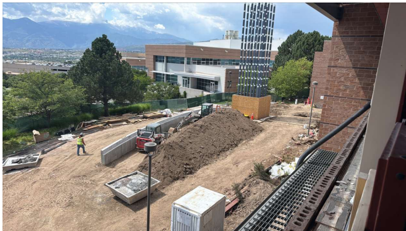
Backfill of the retaining wall for ‘the perch’
