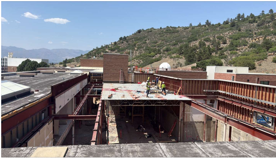
New structural steel and roof framing
